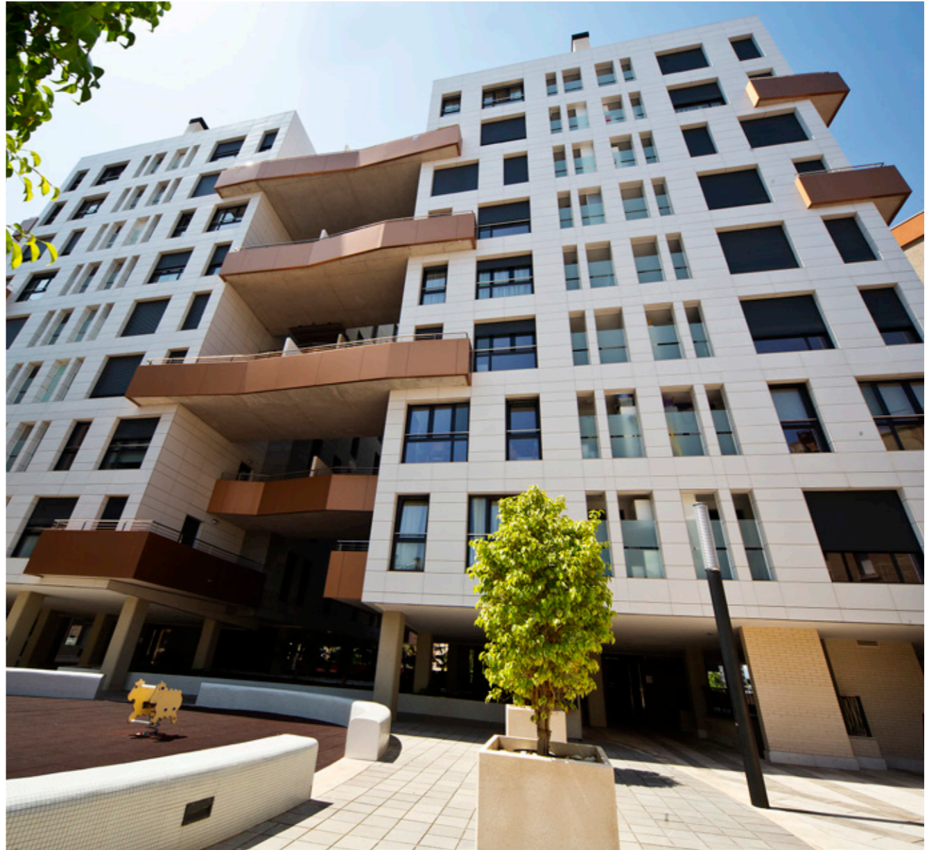
Fachada Ronda Norte Murcia - Spain Keraben Contract & Systems
